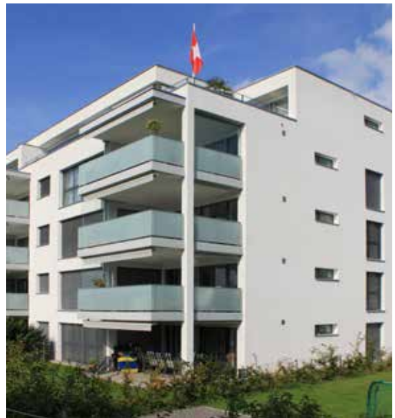
Lotissement Sternmattli, Bollwil ext.: FIXITherm.eps 160 mm; int.: Fixit 341, Fixit 180, Fixit 148, Fixit 770
